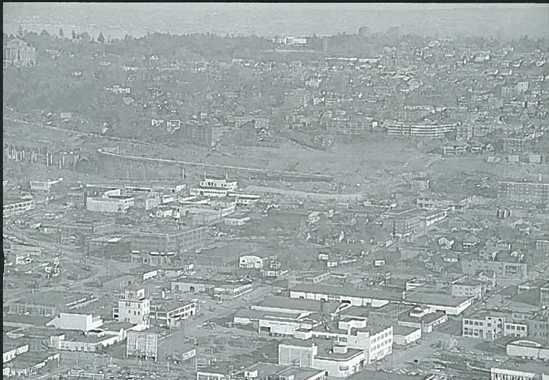
Interstate 5 Construction as seen from the Space Needle, view east to Mercer Street and Eastlake 1962, courtesy of MOHAI
