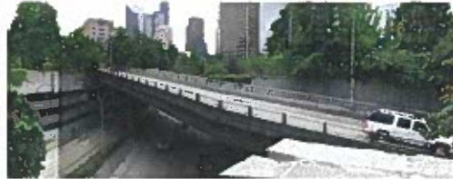
5. 8th Avenue bridge parallel to Freeway Park.
