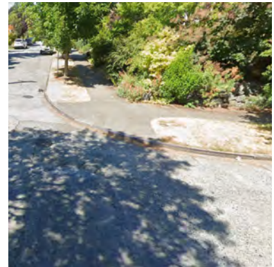
Figure 206. Missing Curb Ramp, NE 44 th St. and 4 th Ave. NE
