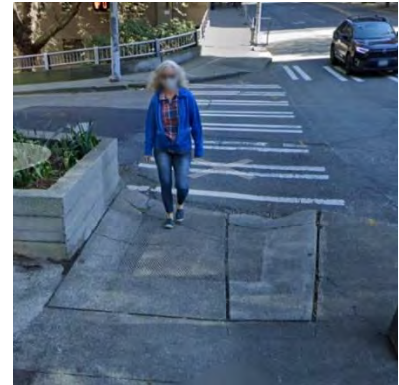
Figure 91. Non-Compliant Curb Ramp, 6 th Ave. and Seneca St.
