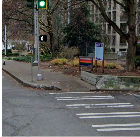
Figure 108. Non-ADA-Compliant Curb Ramp, Seneca St., and Hubbell Pl.
