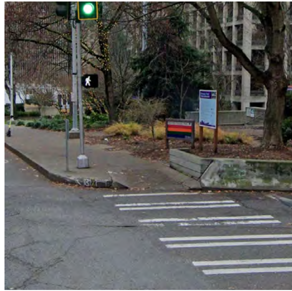
Figure 127. Non-ADA-Compliant Curb Ramp, Hubbell Pl. and Seneca St.
