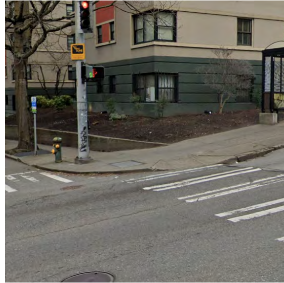
Figure 32. Non-ADA-Compliant Curb Ramp, James St., and 8 th Ave.
