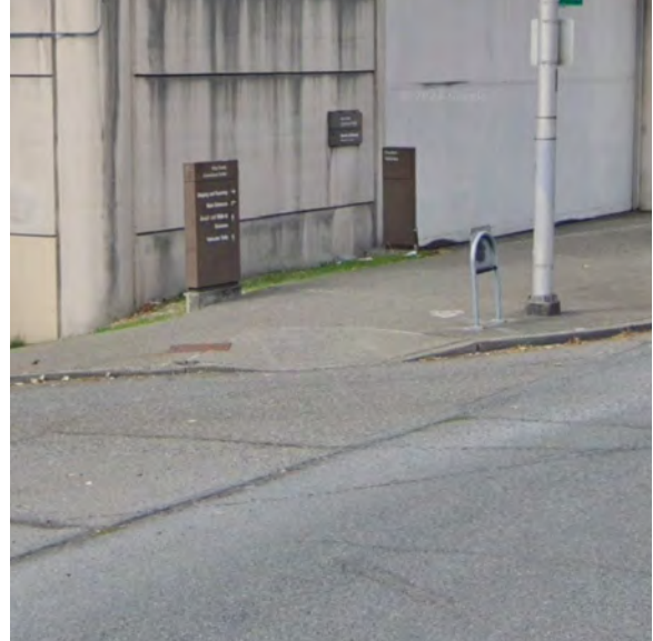
Figure 12. Non-ADA-Compliant Curb Ramp at Jefferson St and 6th Ave.
